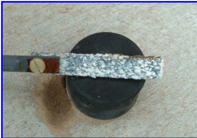
White Rust on Zinc Corrosion Coupon
