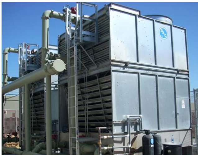
Typical crossflow cooling tower installation
