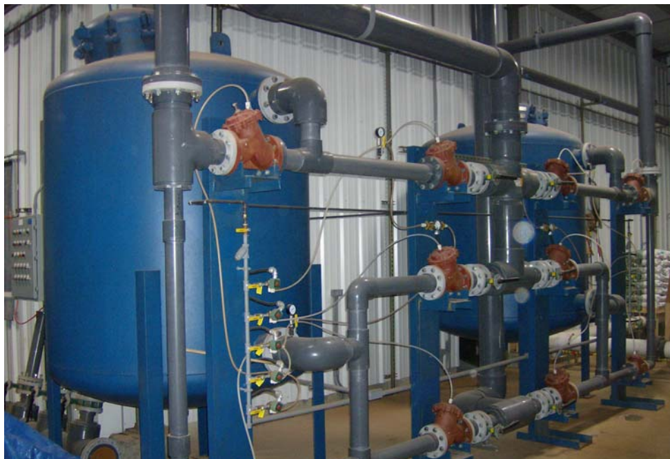
400 gpm dual tank multimedia filter - PLC controlled as manufactured by ProChemTech
